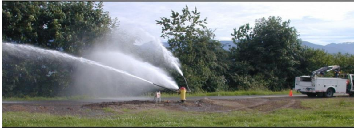
Figure 16: Hydrant Flushing
