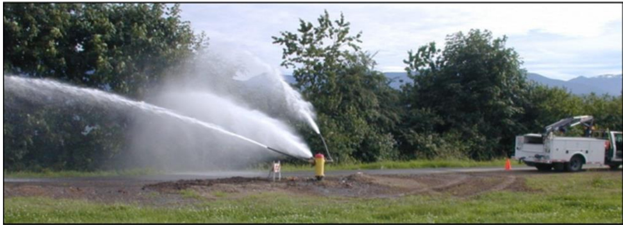
Figure 16: Hydrant Flushing
