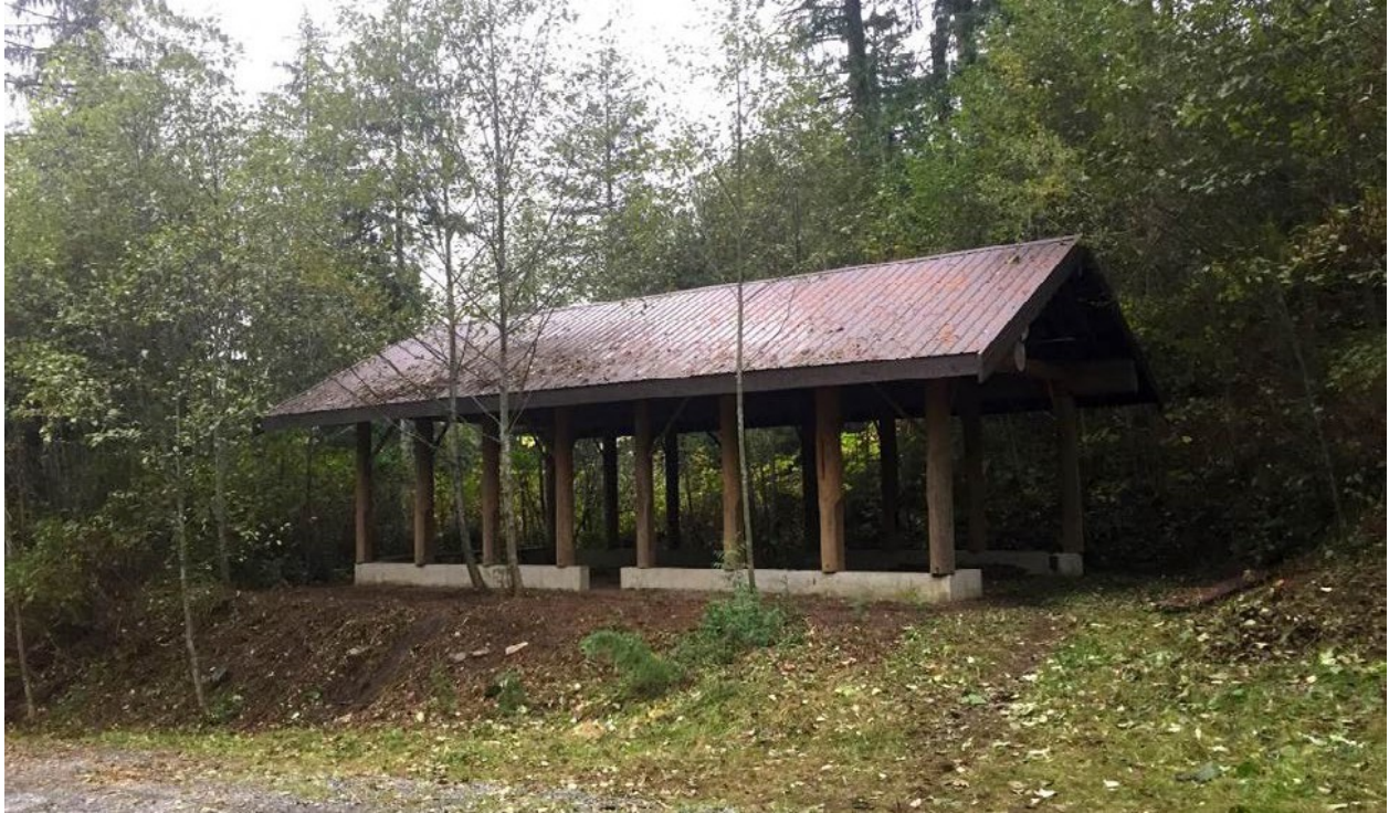
Community Forest: Log Building at Parking Lot (Image © City of Chilliwack, 2015)
