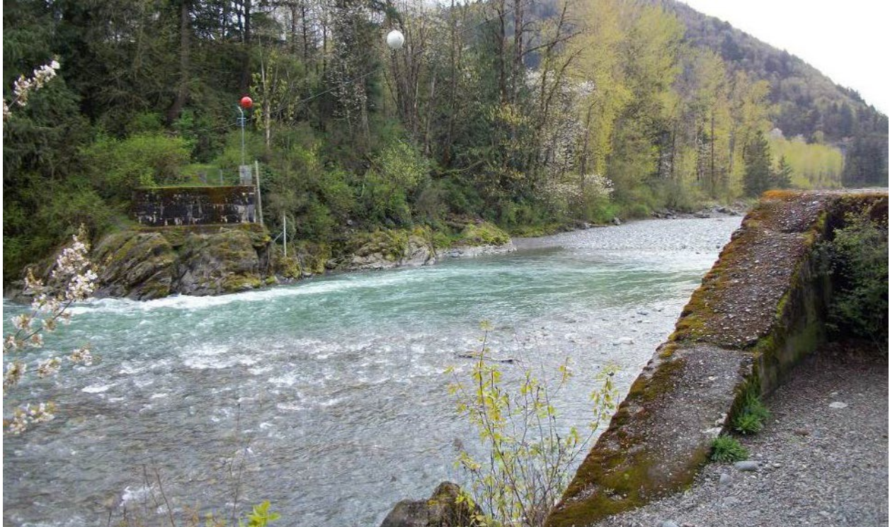
Remaining Abutments of 1910 Bridge (Image © City of Chilliwack, 2017)
