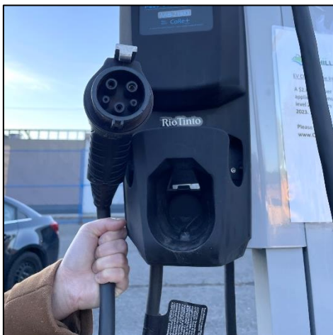
Level 2 Charging Station with a J1772 Connector.
