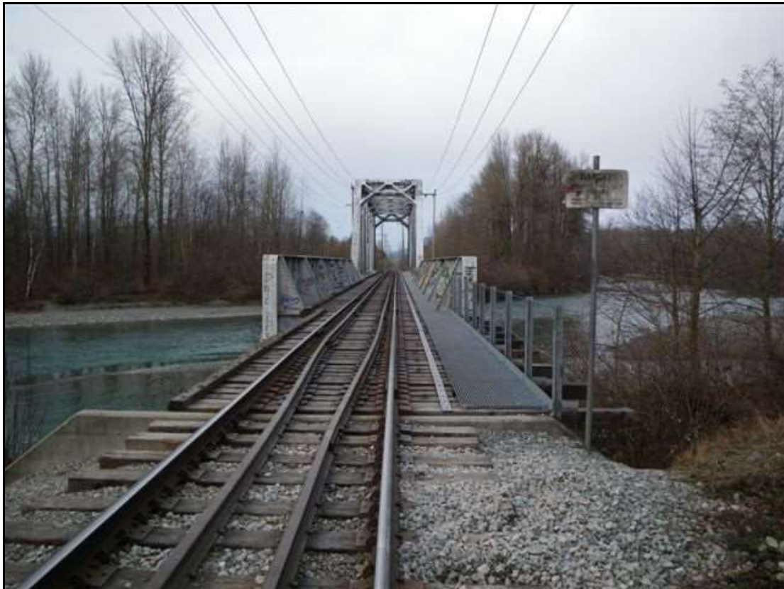
Existing Southern Railway Bridge
