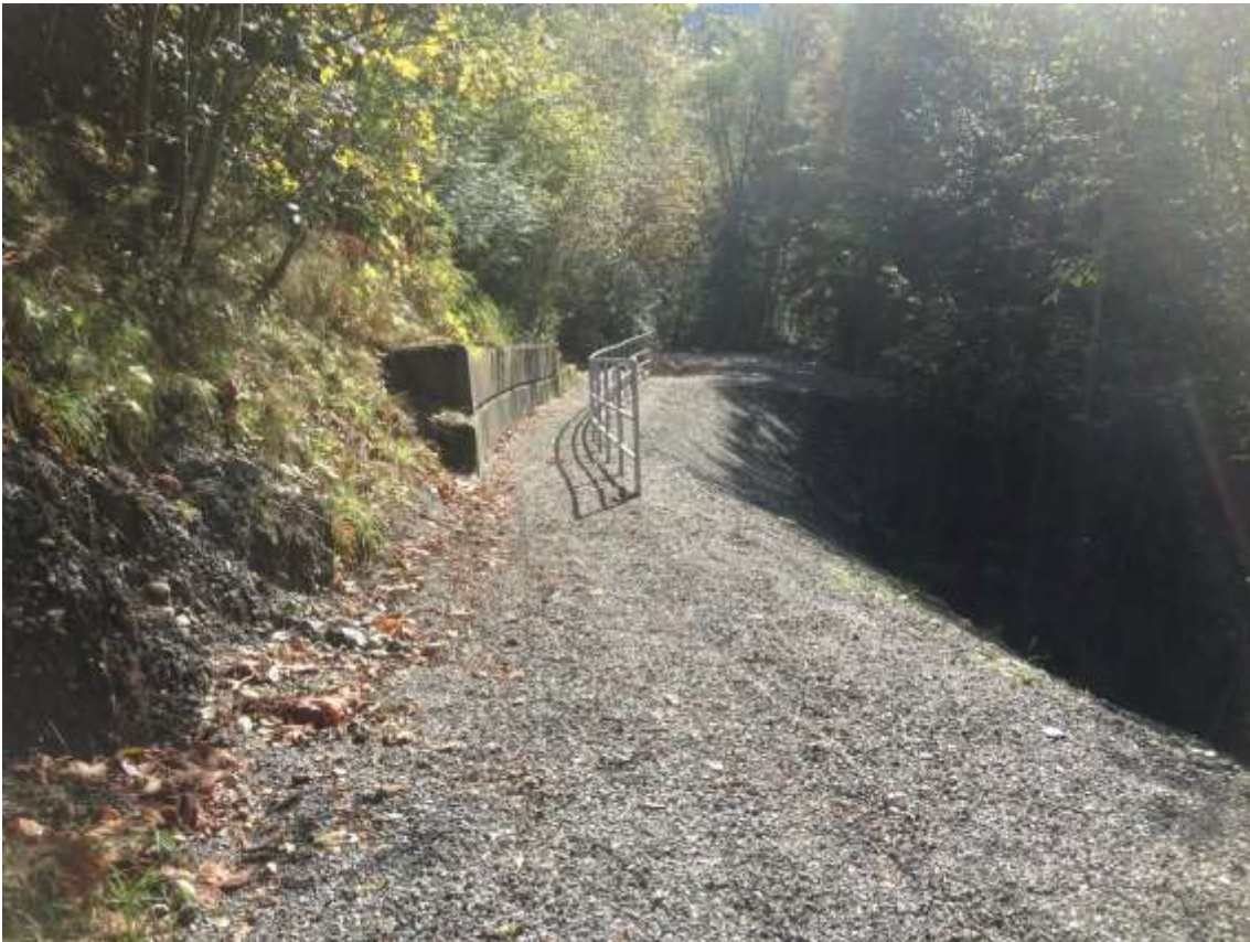
Existing Condition - Marble Hill Trail
