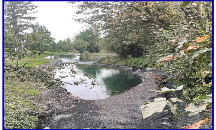
Elk Creek sediment trap following excavation - August 2024
