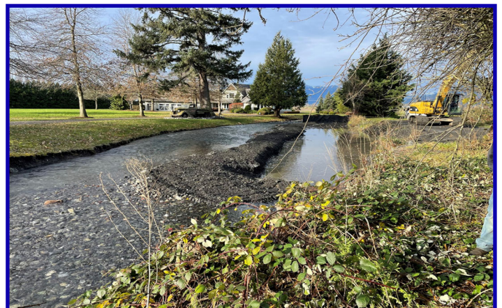
Elk Creek sediment trap following urgent flood prevention works with restored capacity at right bank - December 2024
