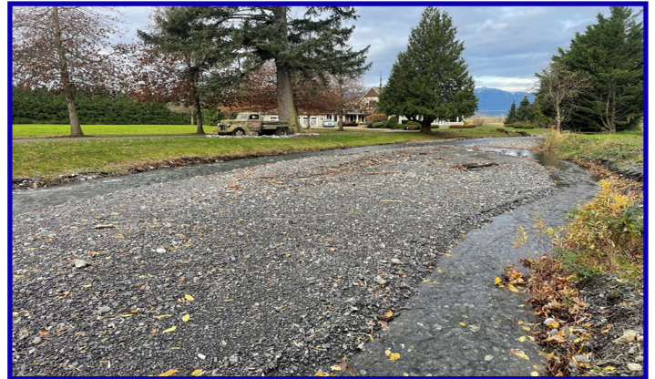
Elk Creek sediment trap prior to prevention works. Note trap has been infilled to capacity by autumn rain events - November 2024
