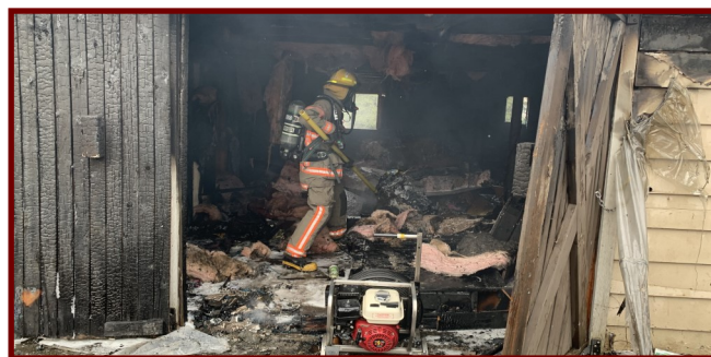
Structure Fire, Broadway February 2024
