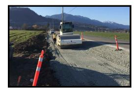
Detailed design was completed including coordination with BC Hydro, Telus and Shaw for necessary relocations. Some portions of the road widening works including base gravels were completed. Continuation of the works will be scheduled once BC Hydro and Telus have relocated their poles during the third quarter.
