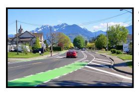
Cycling improvements along these two corridors connecting to the Valley Rail Trail have now been completed. The scope of work involved asphalt rehabilitation, roadway markings, delineators, signage changes and traffic signal improvements. Council's support for this project resulted in Chilliwack residents who worked for the prime contractor to safely continue working during the early stages of the pandemic.
