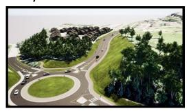
Works include one single-lane roundabout, approximately 250m of new road construction, storm main relocation, drainage works, streetlighting and trail connections. This new connection to Teskey Way will reduce travel time for residents on the east side of Promontory and will reduce traffic volumes at the intersection of Teskey Way and Jinkerson Road/Hudson Road. The road will be constructed within the existing Ross Road right-of-way. Construction is scheduled March 2021 to September 2021.
