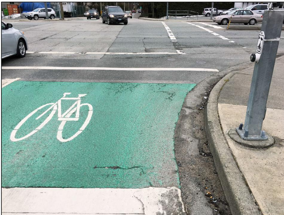
Figure 5.12 – Bicycle detector marking (Boulder)
